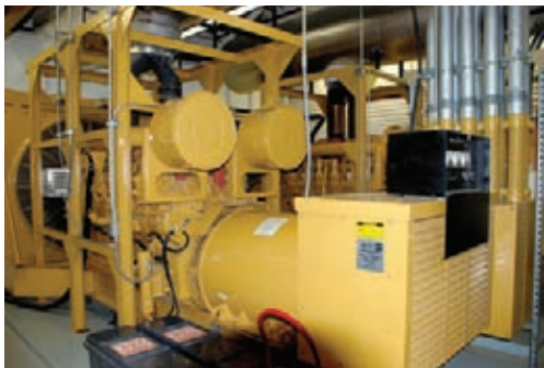
Emergency power supply system (EPSS).
